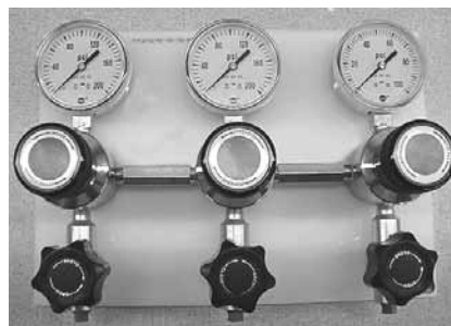
three-regulator panel - inlet may be from the left or right
